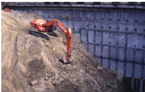
(c) Excavation in Progress
