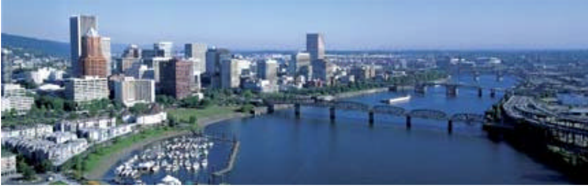
Fig.1 The city of Portland seen from the Willamette River
